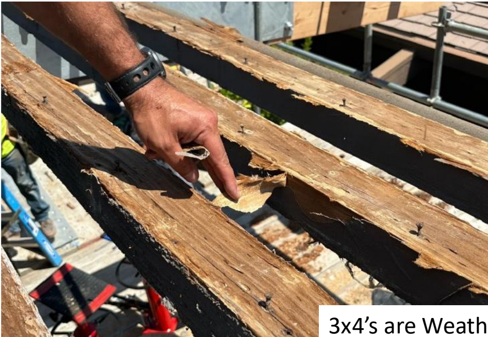
Plywood is Soft and Delaminated
