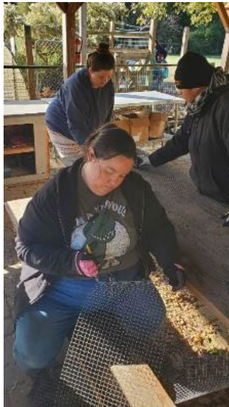
Figure 151. Cutting wire mesh for planter boxes.
