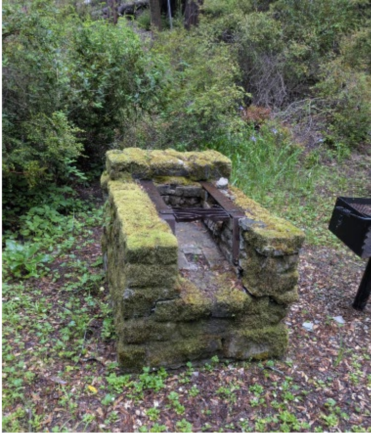
Figure 48. Example of an original fireplace at the Memorial Park Campground is on the Pescadero Creek in San Mateo County (photo provided by Tom Waschura, April 2025).
